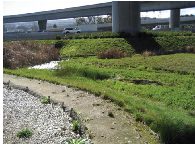
Stormwater runoff from a small area at the Airport flows into bioswales before being discharged to a wetland area.
