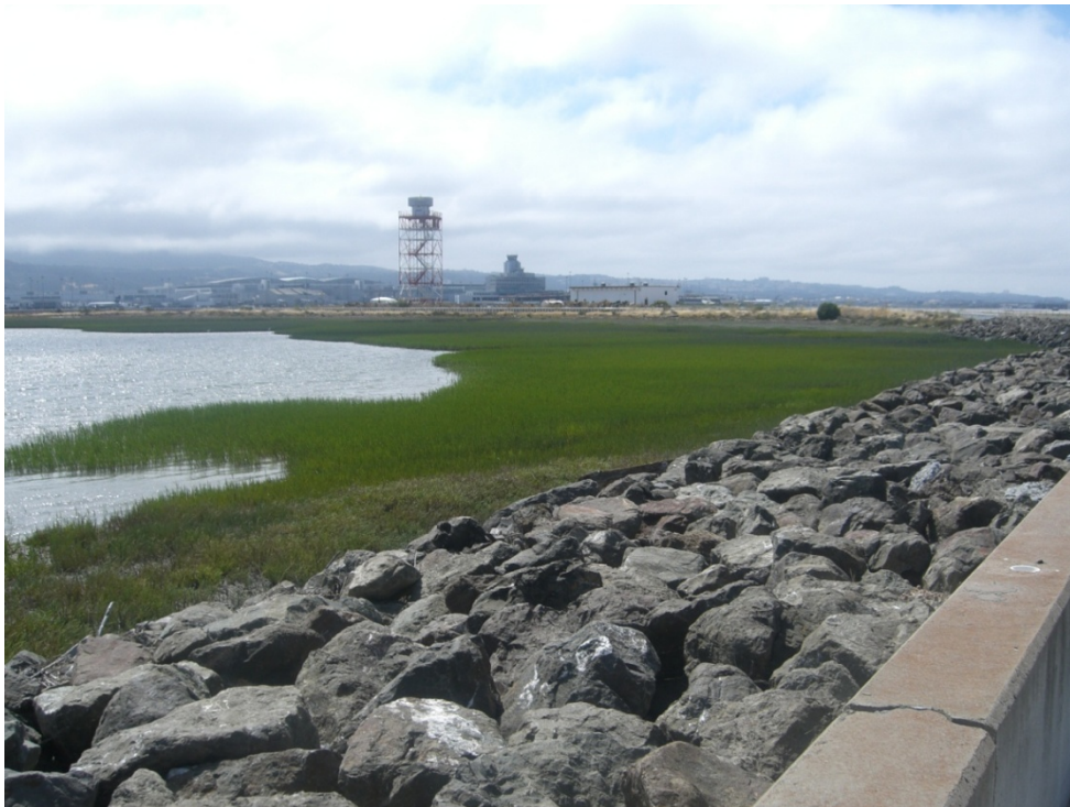
Photo 2. Rip-Rap and Tidal Marsh
